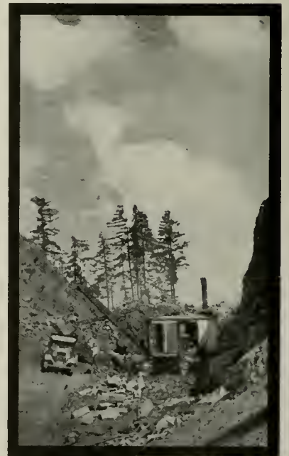
Fisher Brothers cut 100 feet through solid rock and moved 73,000 yards of dirt to complete their contract on the new Pacific Highway between Portland and Salem
